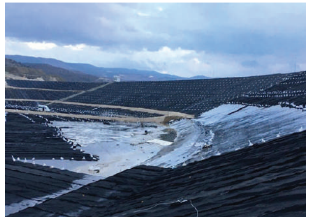
An impermeable layer was created in the mining waste site using Bentoshield..
