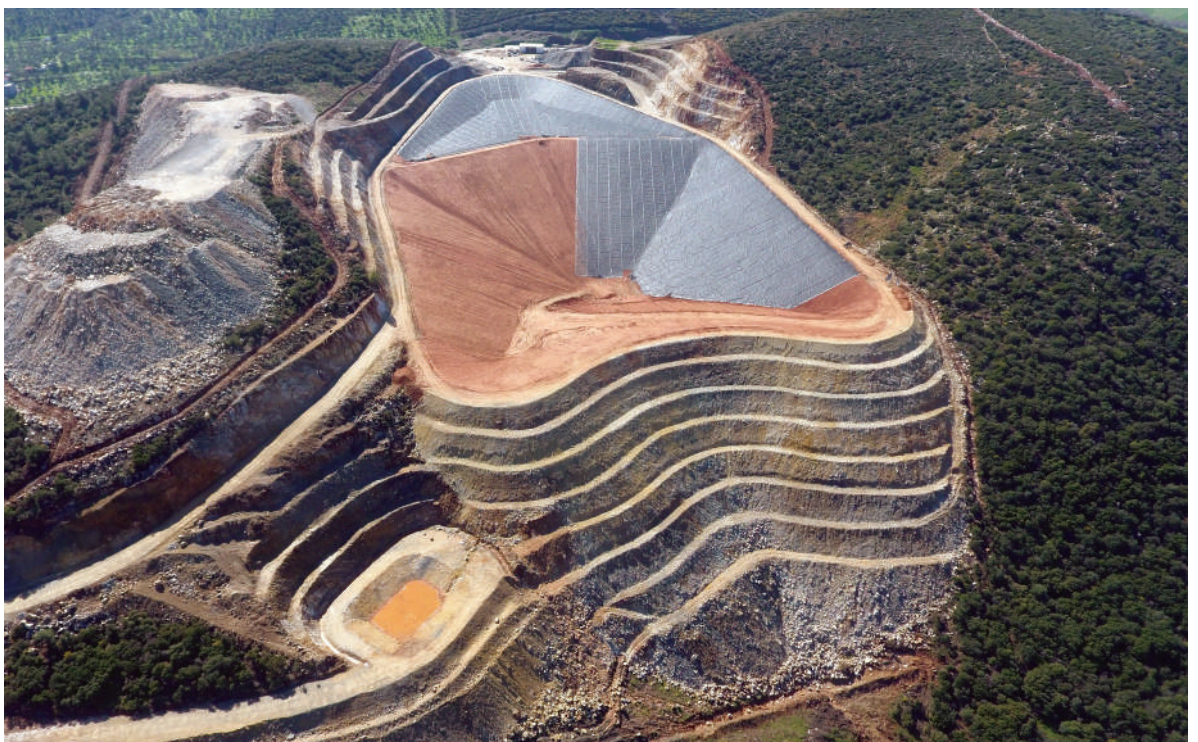
An impermeable layer was created in the mining waste site using Bentoshield..
