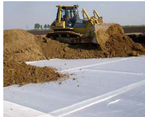
Tectgrid and Tectex soil reinforcement and separation in road structures
