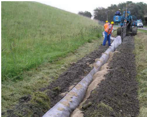
Geodrain and Tectex drainage system in road construction
