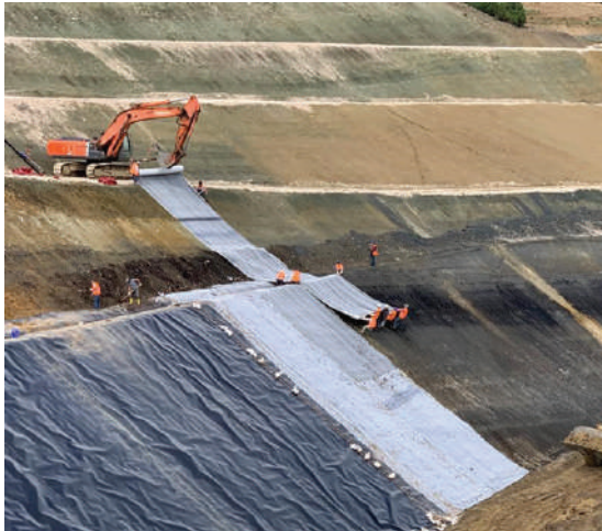
An impermeable layer was created in the mining waste site using Bentoshield..
