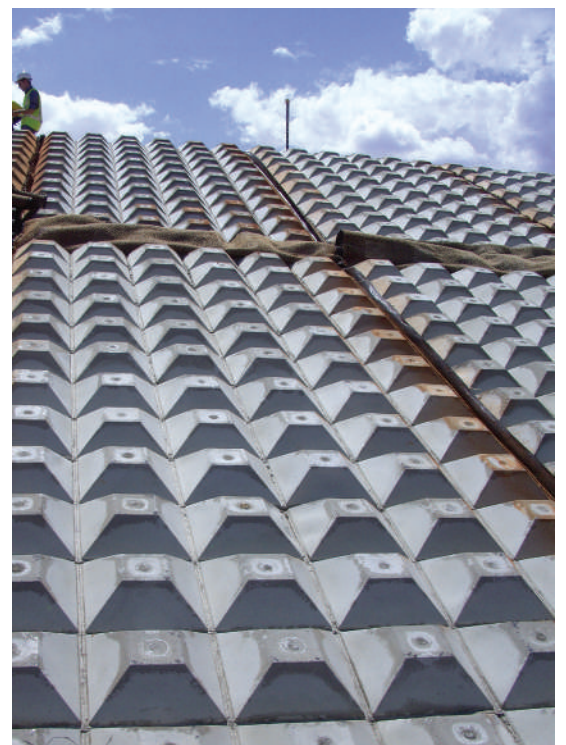
Erosion control with TechFlex in the Roy Hill project.
