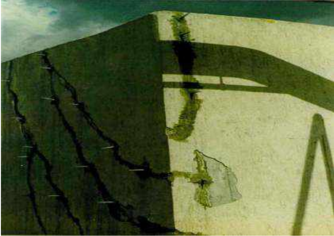
EPOXY İLE STATİK TAKVİYE
